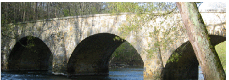
Booth’s Bridge, Antietam Creek, Maryland.
